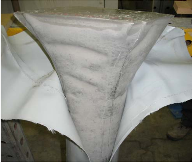
Figure 9: Demoulding of the fabric formed concrete column.
