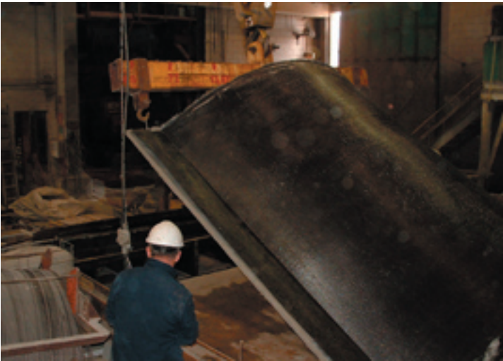
3. The resulting funicular shell is inverted to make a mold for precast production.
