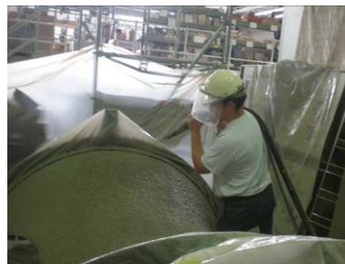
Fig. 9: Shotcrete application
