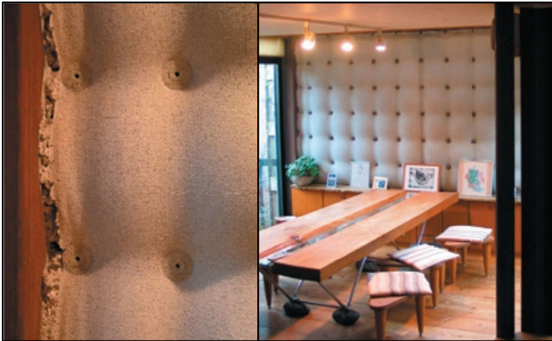
Figure 6. Quilt-like formwork pattern used for the Eiji Hoshino Residence (Mark West photos).
