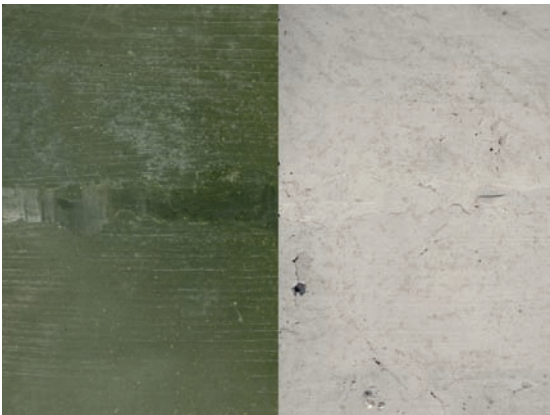
Figure 15: Joint of adjacent wax elements sealed with hot wax (left). Concrete surface cast against wax surface with sealed joint (right).
